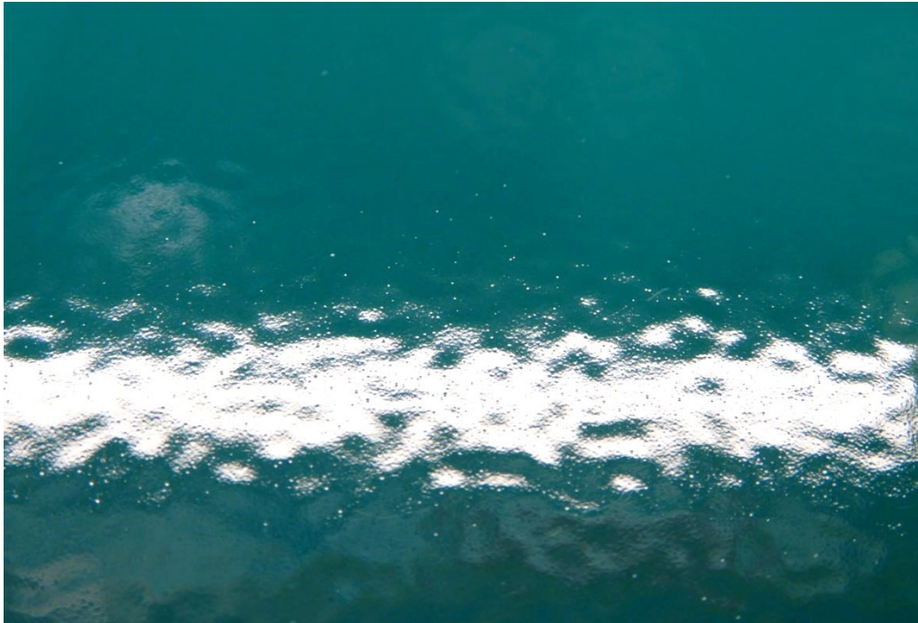
Figure 1: P1-1 initial state (micro blisters / pinholes)
