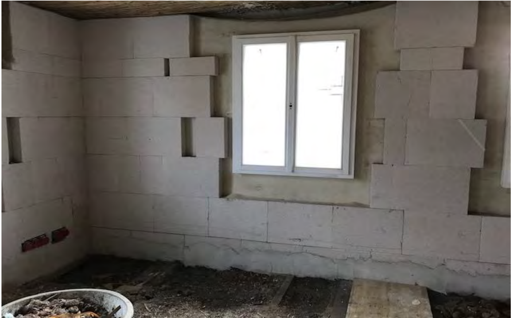
Mineral foam insulation (living rooms)
