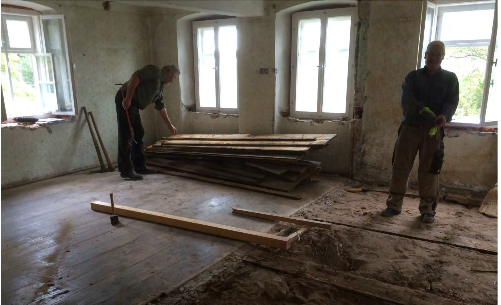
Kitchen during renovation
