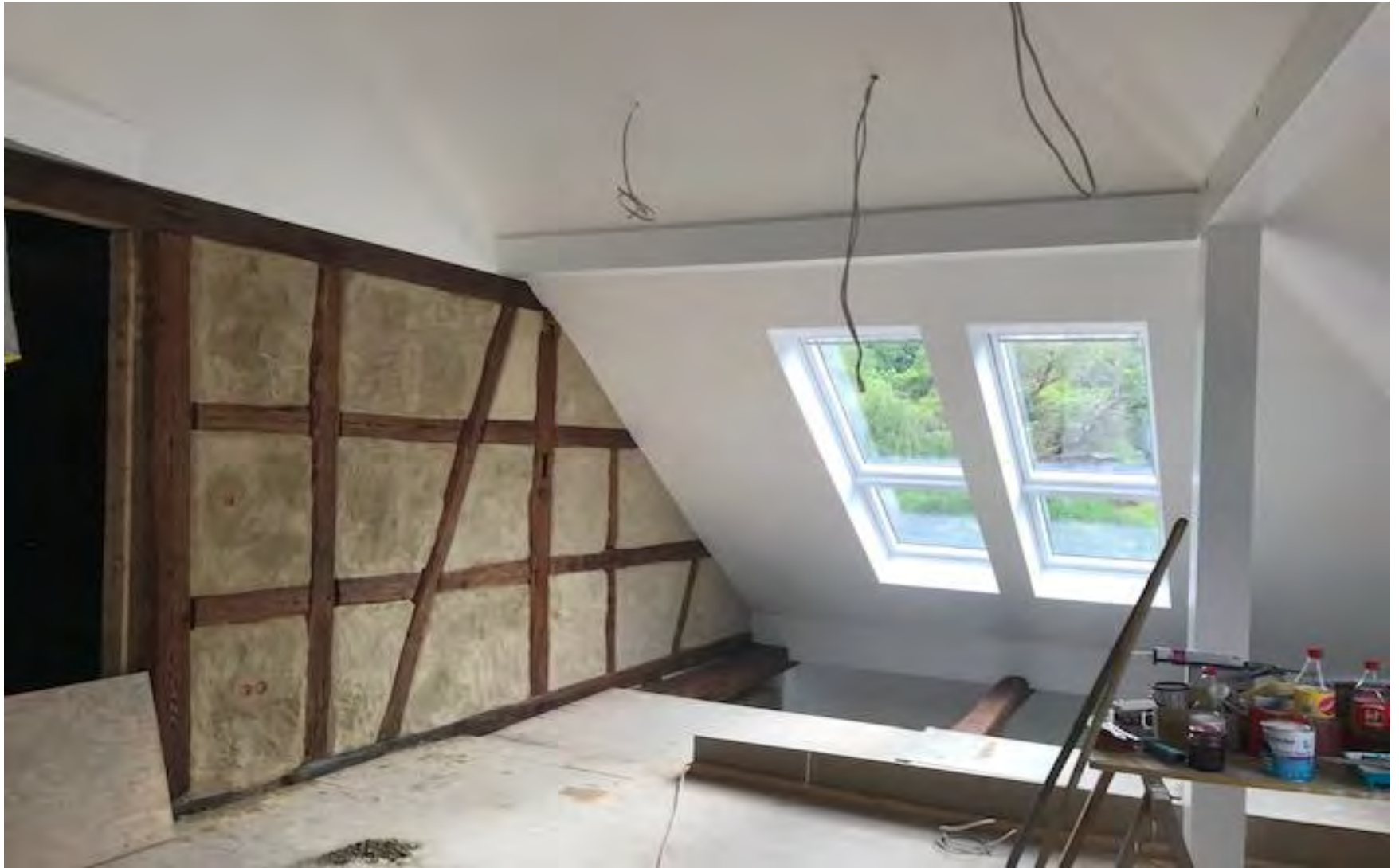
Office rooms during renovation
