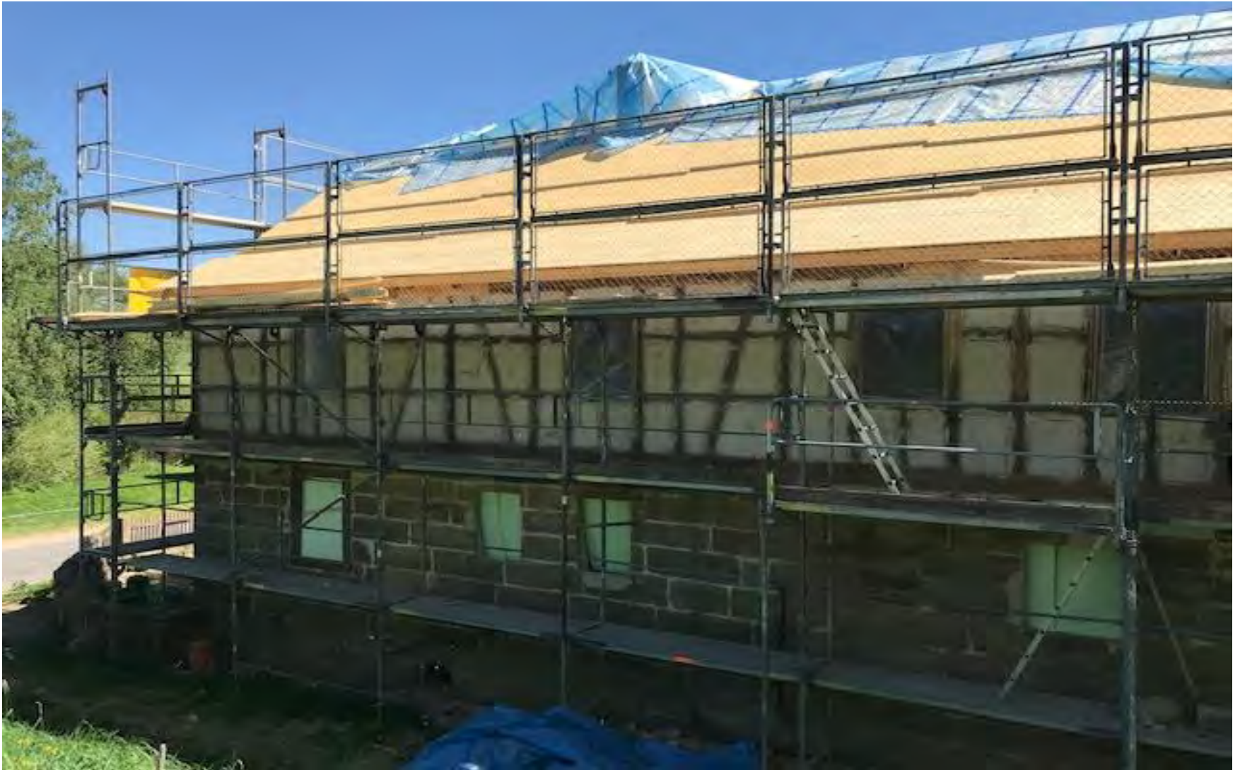
Renovation of the roof and the facade
