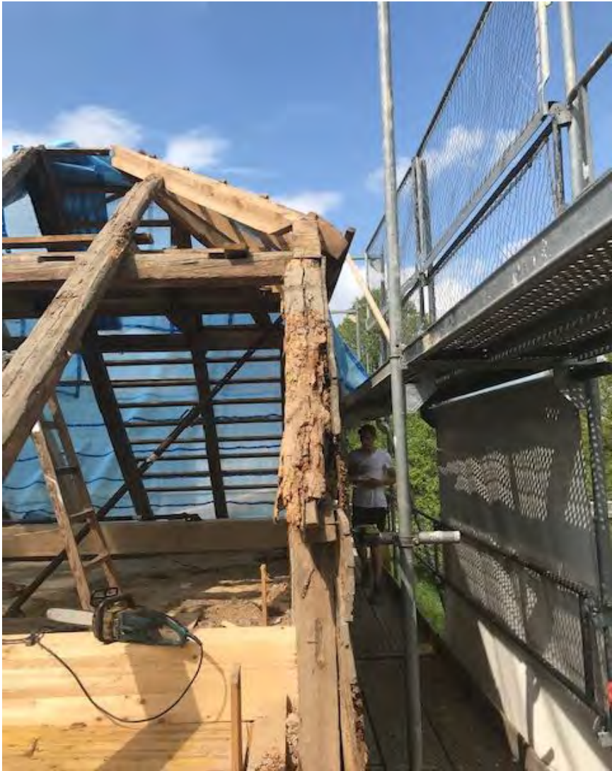
Major damages of the roof structure
