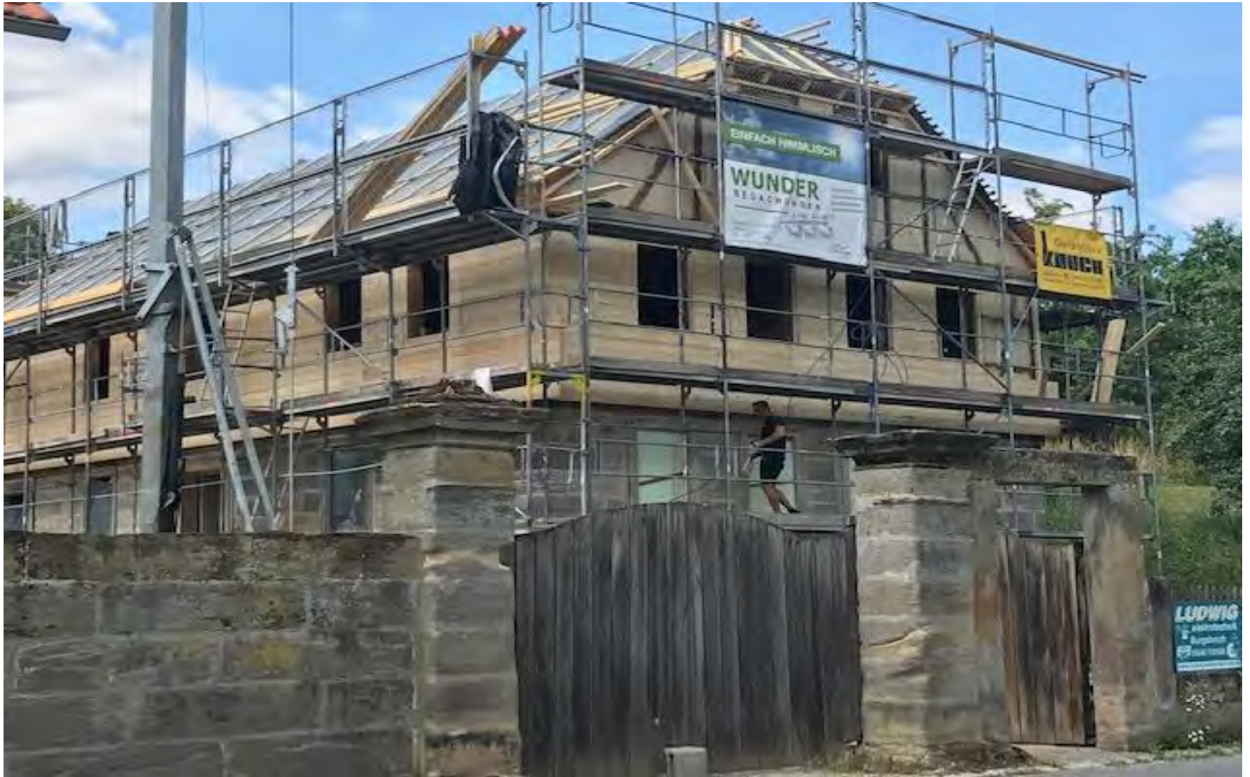
Renovation of the roof and the facade
