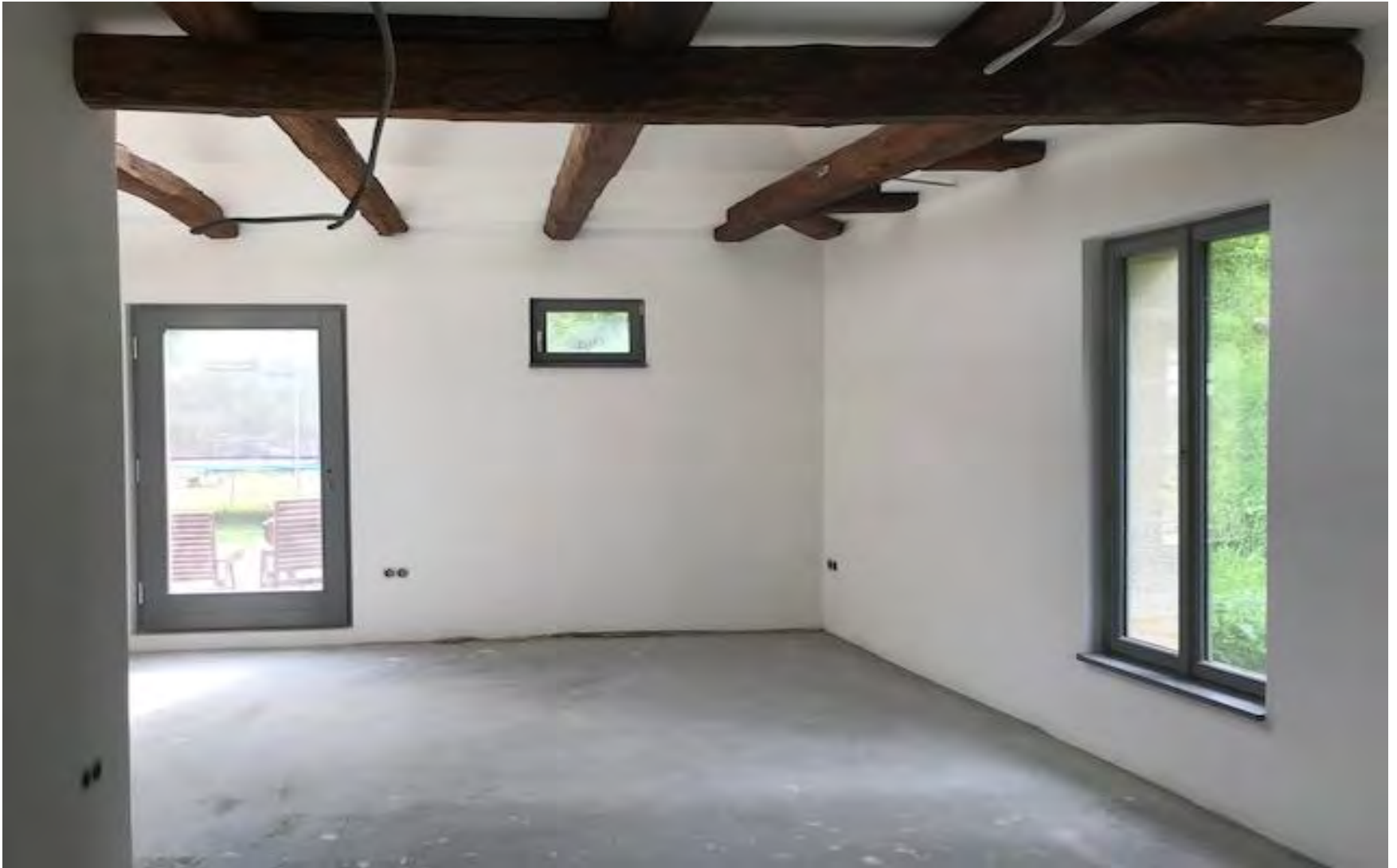
Office rooms during renovation
