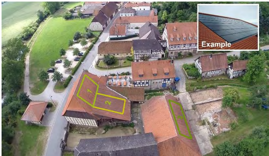
Image 5: Photovoltaic concept in cooperation with the monument protection authority
