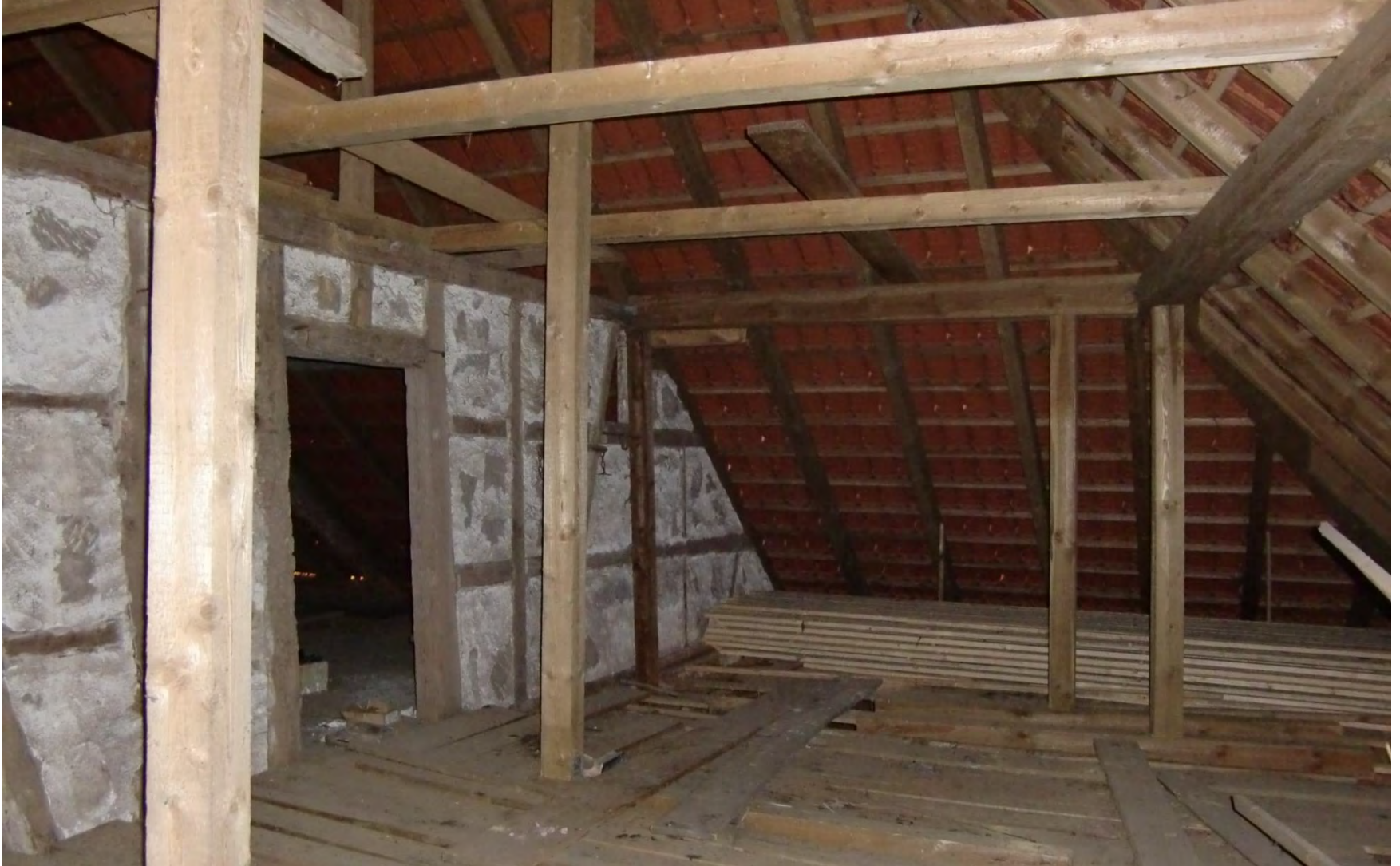
Office rooms before renovation
