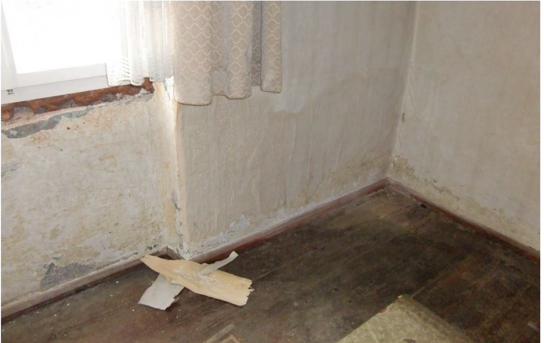
Kitchen before renovation
