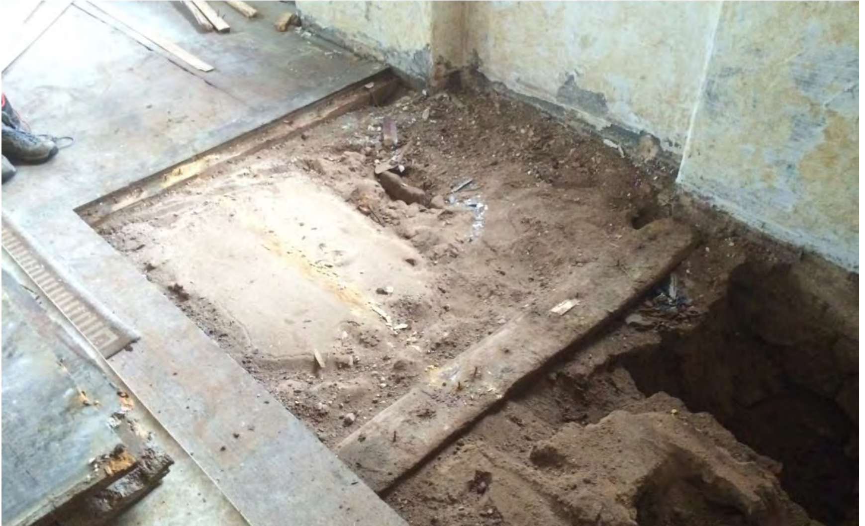
Kitchen during renovation
