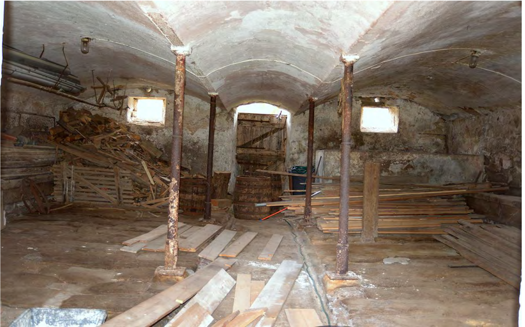
Seminar rooms before renovation
