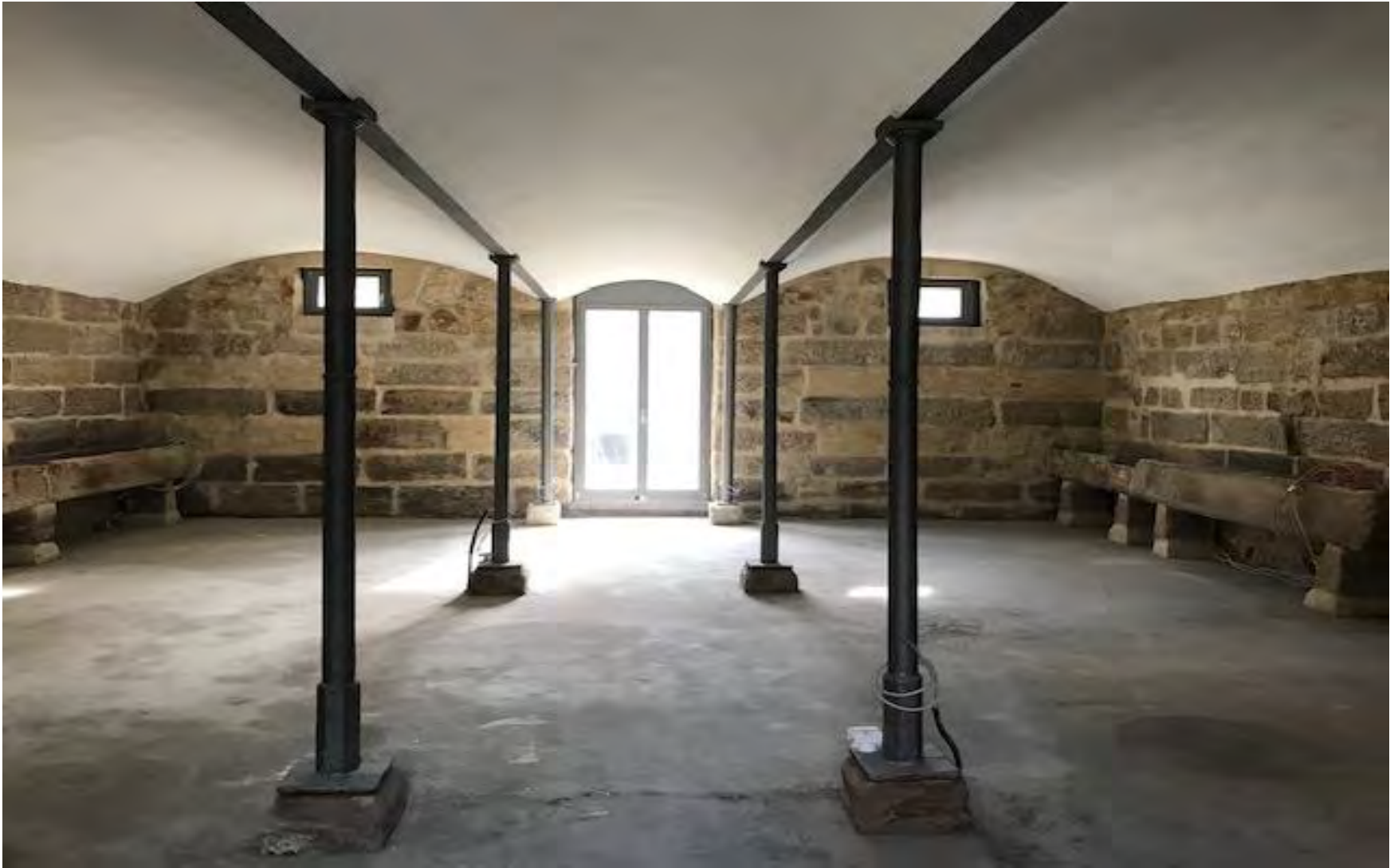
Seminar rooms during renovation
