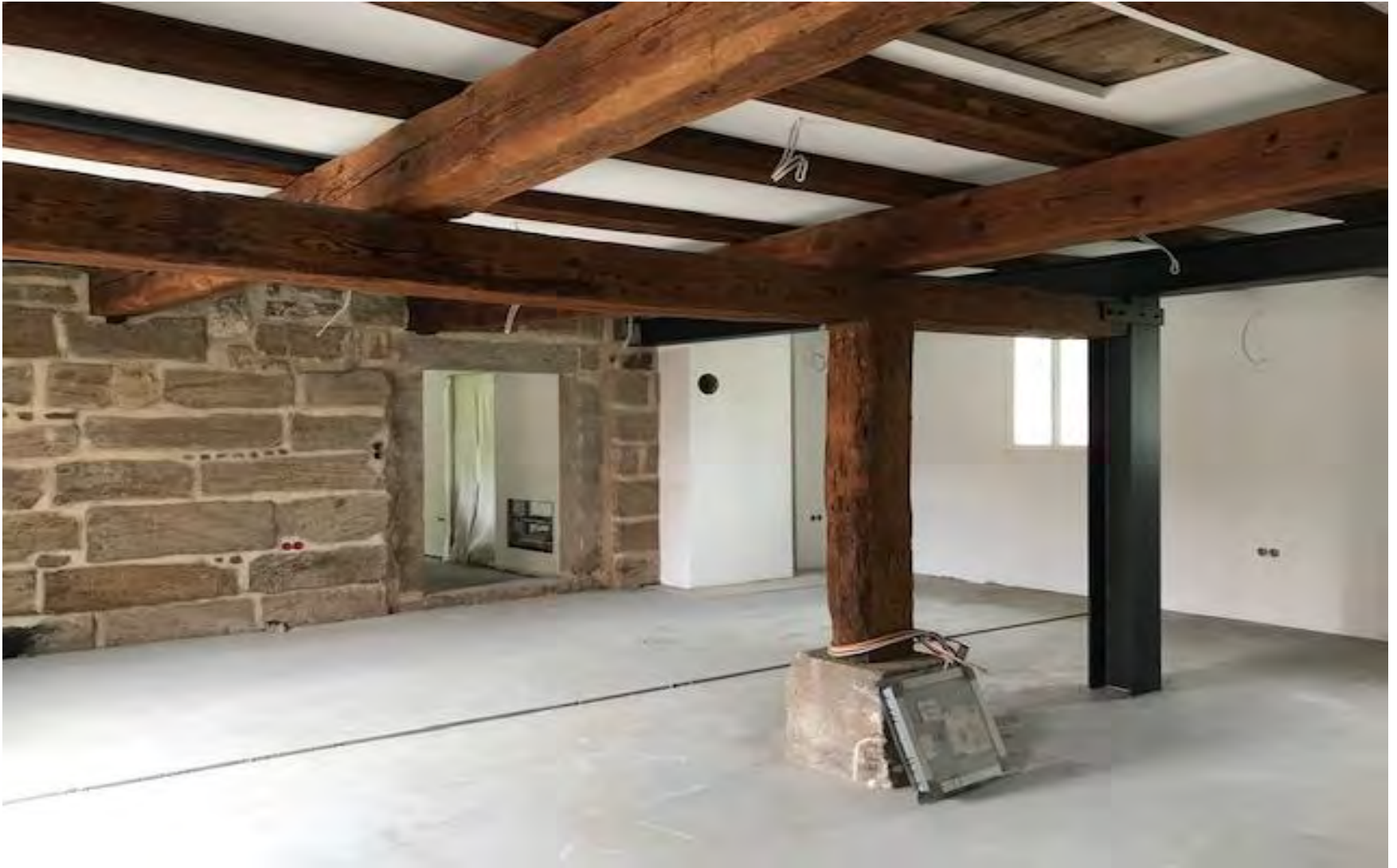
Living room during renovation
