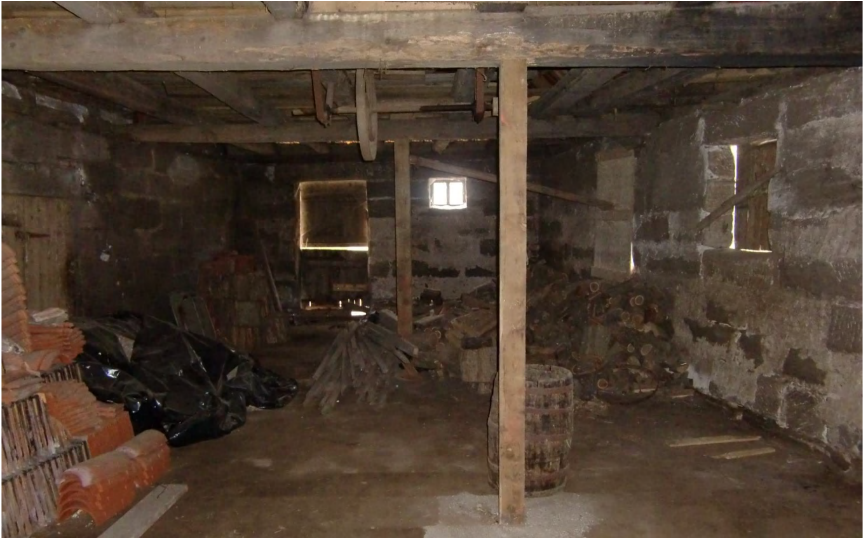
Office rooms before renovation
